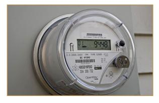
The all-digital meter or smart meter measures the use of electricity and stores and reports that data
